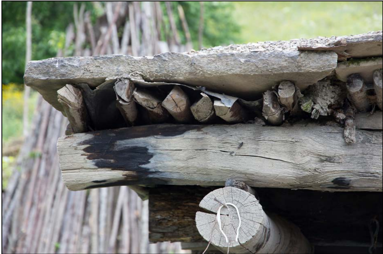
Figure 51. Traditional Khevsureti home of Gaga Arabuli, Barisako village, Khevsureti, Georgia. Roof detail of oak-poplar frame with schist tiles.
