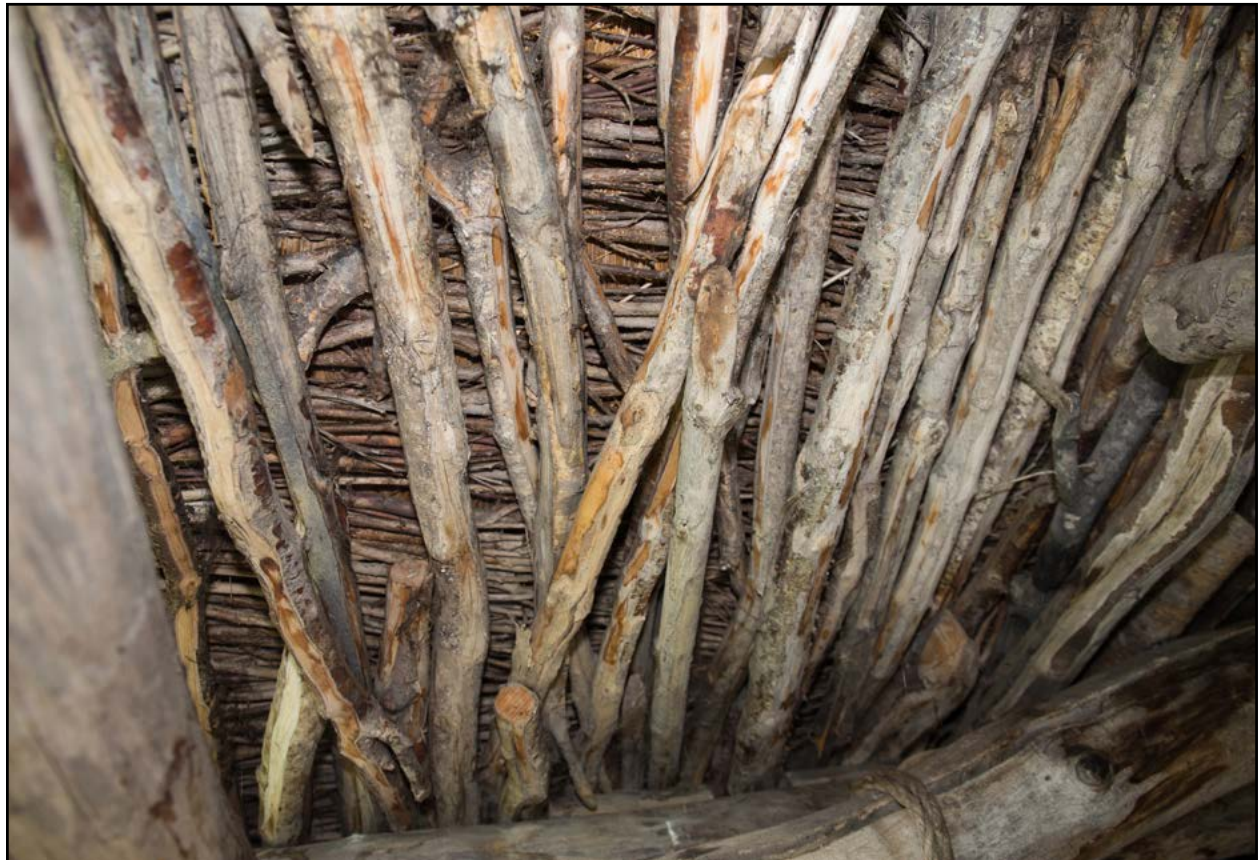
Figure 53. Interior of Gaga Arabuli's home, Barisako, Khevsureti. Roof detail with Rhododendron luteum Sweet webbing above oak and poplar frame.
